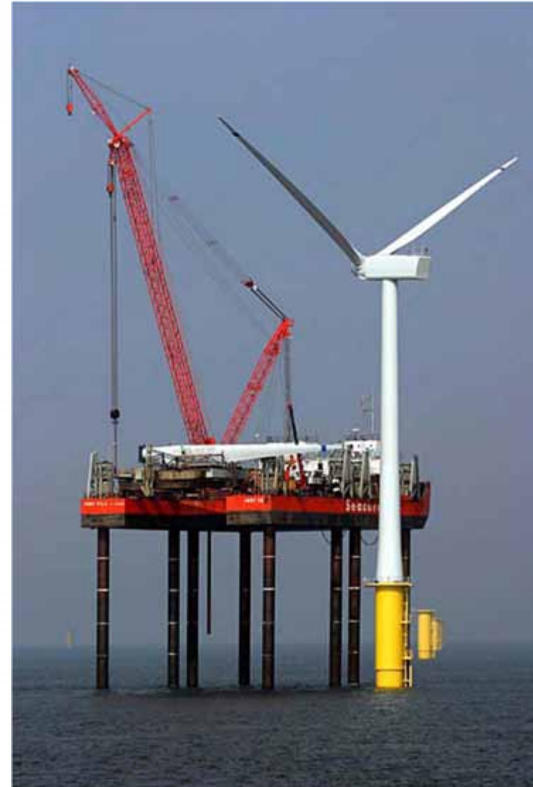
Offshore wind turbine under construction
